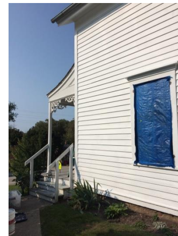
Summer 2017 Shutters Off, During Painting
